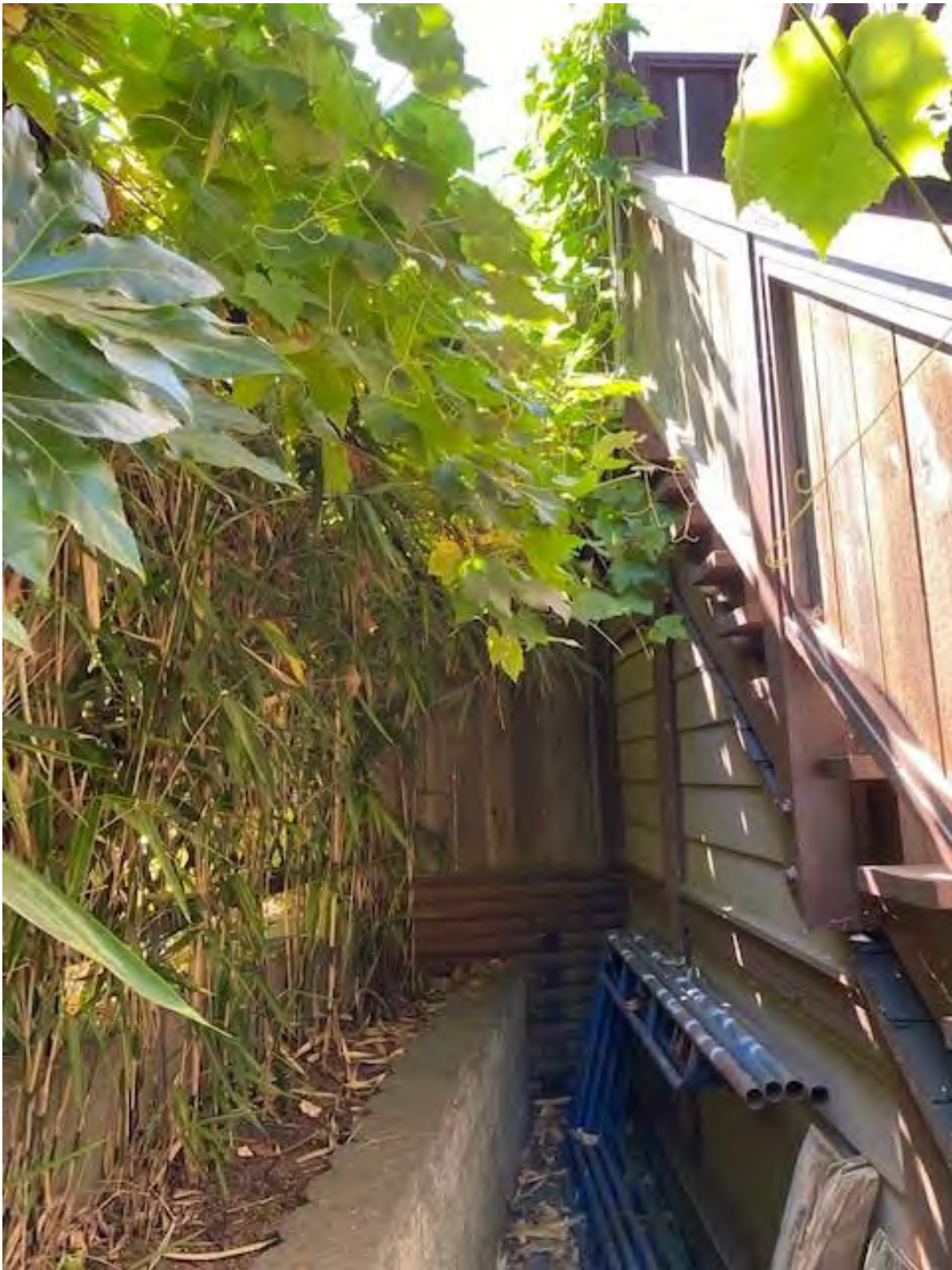
Figure 4: Image of Existing Staircase
